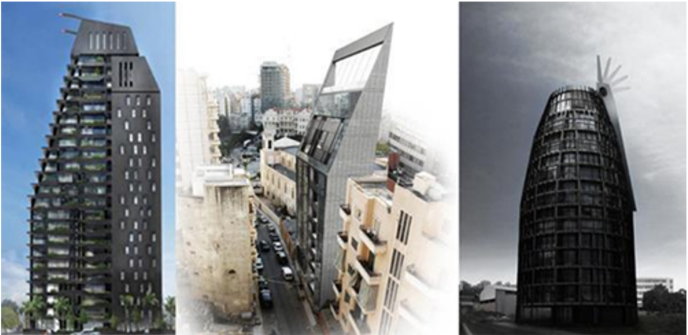
Buildings under construction in Beirut, with a triangular or conical ending. Architect: Bernard Khoury. Source: bernardkhoury.com
